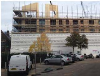
On Bacton Low Rise, a 294 flatted scheme constructed by Rydon Construction Ltd, we are using Cross Laminated Timber for the construction of 44 residential flats for LB of Camden. Phase 1 completion is set for March 2015.
