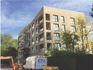
The use of cross laminated timber for the construction of Phase One of our scheme at Bacton Low Rise for Rydon Construction Ltd has allowed quick progress with only internal fixtures and balconies for Block A remaining. The three phase development in LB Camden consists of a mixed tenure of 294 flats.
